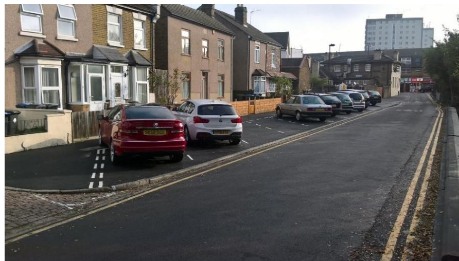
Figure 9: Widening works at Gilbert Street
