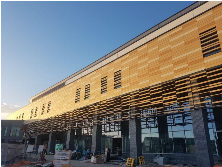
Figure 5: Redevelopment of Chase Farm Hospital
