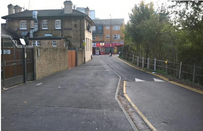
Figure 14: Improvement works at Gilbert Street
